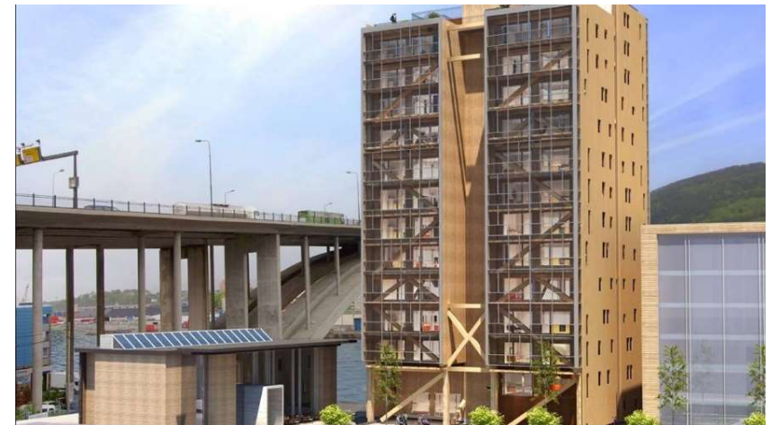
'Treet' – Currently the World's second tallest timber (hybrid) high-rise building, in Bergen, Norway
