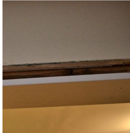
Typical sample of a linear seal surrounding a fire rated door
